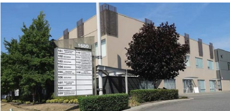
1680 BROADWAY STREET PORT COQUITLAM, BC
