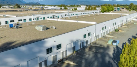
1525 BROADWAY STREET, PORT COQUITLAM, BC
