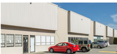
1776 BROADWAY STREET, PORT COQUITLAM, BC
