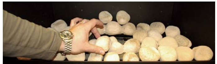
Figure 23.n Place the first Top faux Rock.
