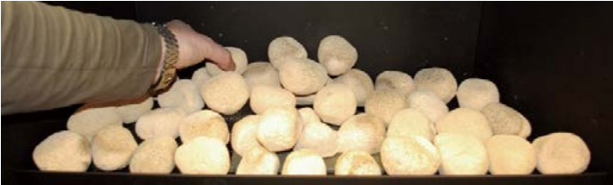
Figure 23.r Place the fifth Top faux Rock on top, behind the pilot assembly cover.
