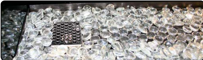
Figure 21.b Completed firestone installation
