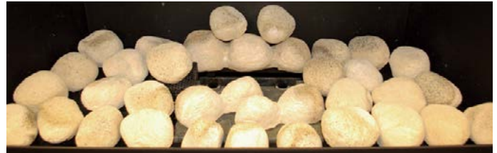
Figure 23.m Completed lower layer of ceramic Rock.
