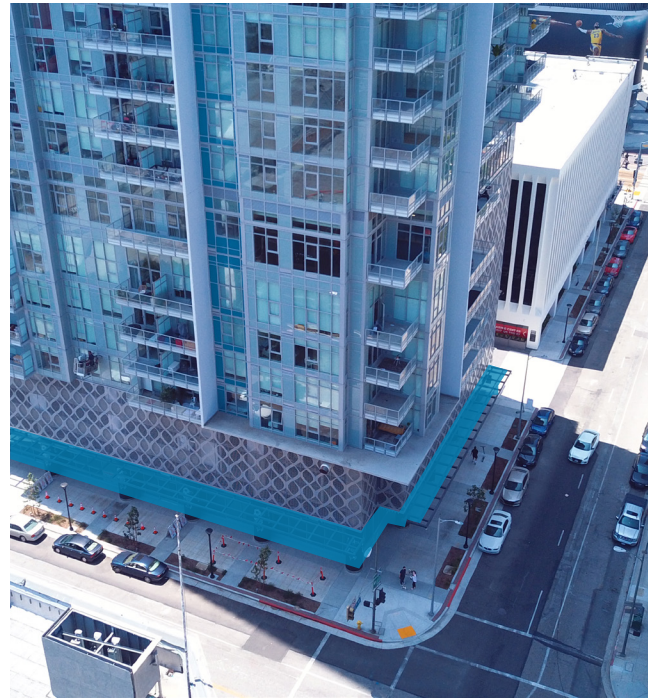
Building C Retail
